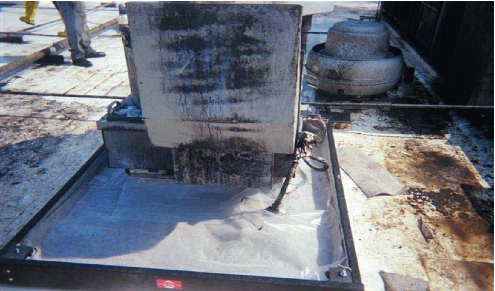
Lay Grease Barrier/Assimilation Pad in unit
