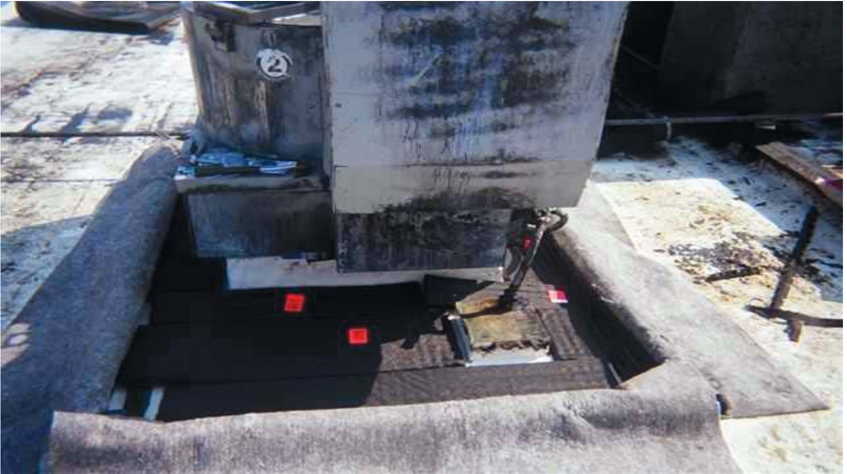
Install Drainage Board with Orange Sticker Up
