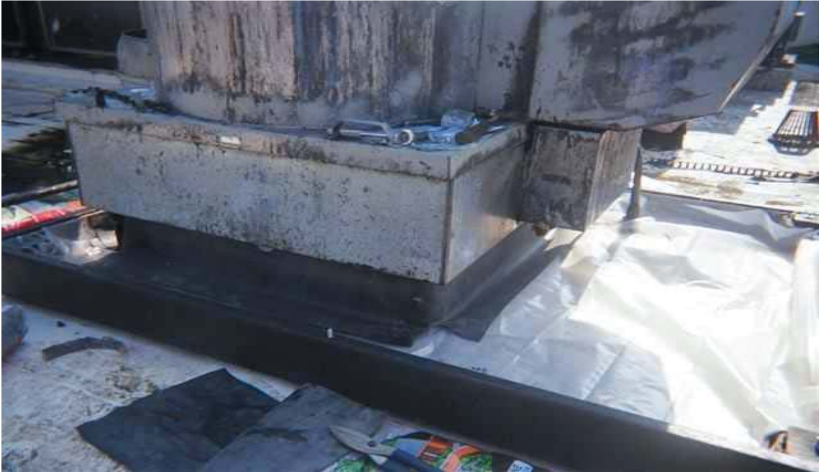
Install Grease Deflector Shield
