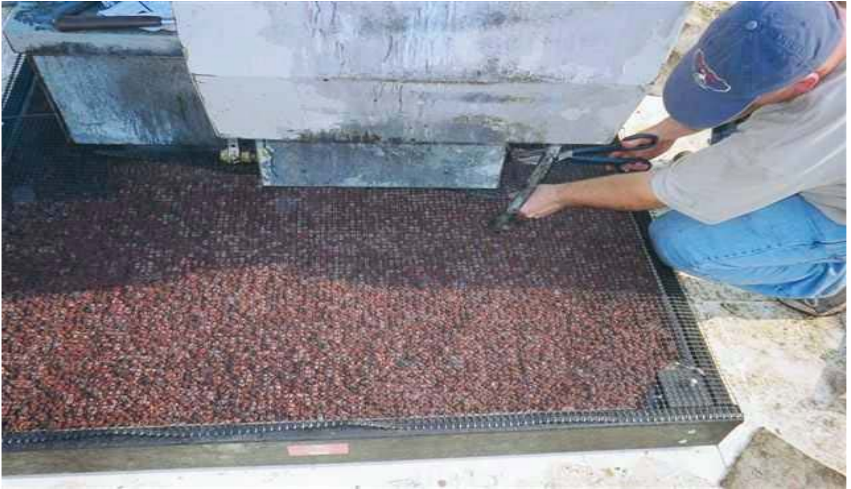
Install Containment Screen
